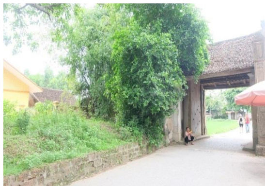
Figure 1. Duong Lam village gate (Source: Author, July 21, 2020)
