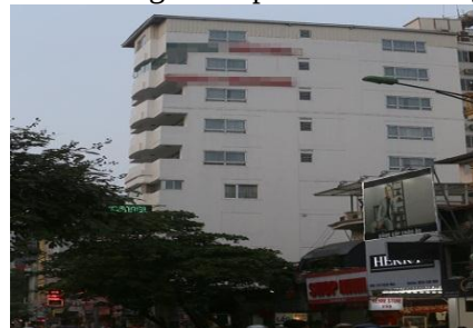
In 2007, the building 221-223 Bach Mai, Hai Ba Trung, Hanoi was built 15 meters over the permit
