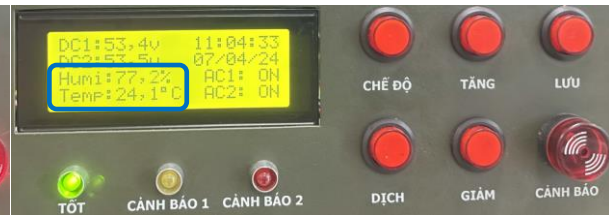
Figure 14. Respond of device when ending temperature and humidity problem
