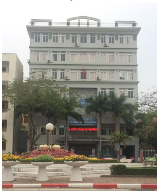
Figure 1. Thai Nguyen Social Insurance Building Thai Nguyen Social Insurance Building is located on the Hoang Van Thu street, the largest administrative center in Thai Nguyen
